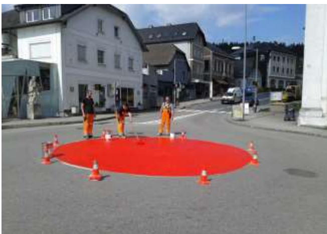
Figure 4. Mini roundabout with a passable central island in the author's place of residence Voecklabruck Hrapović, 2020, prva knjiga
