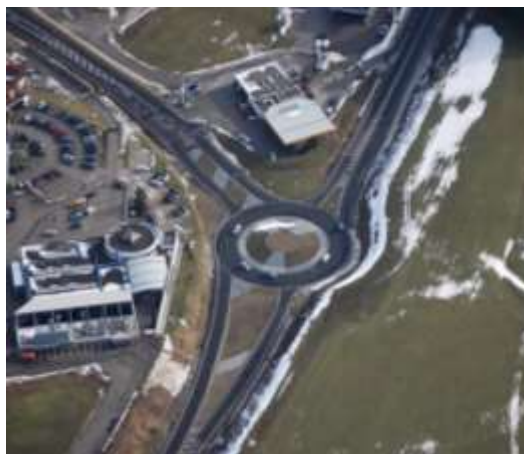
Figure 6. Example for a three-arm roundabout at the intersection of the Austrian national roads B38 /B127 Hrapović, 2020, druga knjiga
