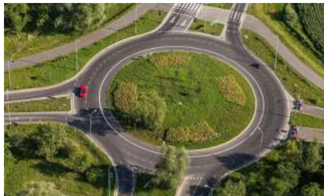
Figure 14. A large 2-lane roundabout Kleine Zeitung, 2016
