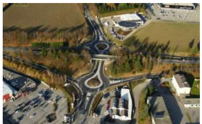
Figure 20. Two smaller roundabouts of the "dog bones" type near Ried im Innkreis Hrapović, 2020, prva knjiga
