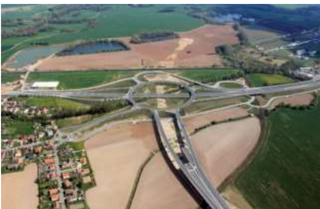
Figure 17. The large roundabout in the Czech Republic near Opatovice Hrapović, 2020, prva knjiga
