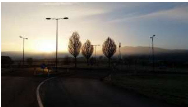
Figure 3. Example for (Three)Tree circle (not traversable): roundabout on the Schoerfling District Road L1265 in Upper Austria Hrapović, 2020, prva knjiga
