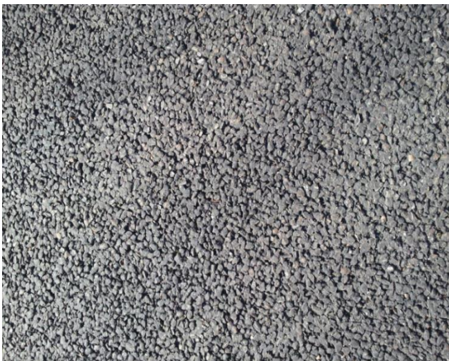
Figure 6. Texture of an SMA 5 LA in Baden-Baden, Germany, Source: F. Garthe, 2014
