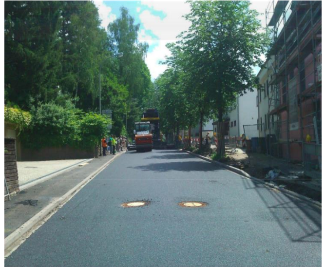
Figure 7. Installation of SMA 5 LA in Baden-Baden, Germany, Source: F. Garthe, 2014
