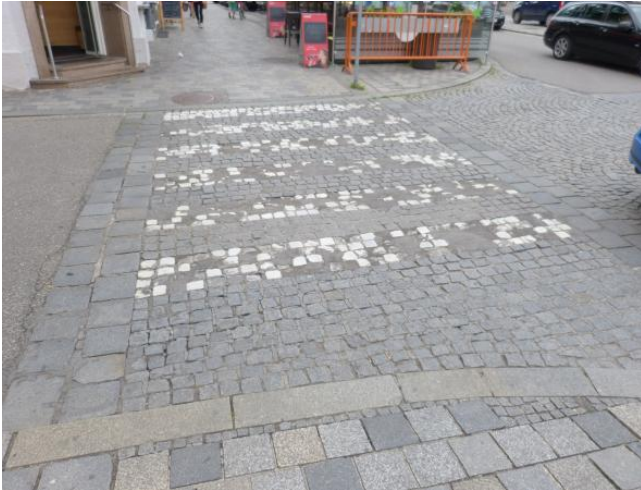
Figure 28. Asphalt-filled patches at a pedestrian crossing made of marble and granite cobblestones Source: Hrapović, 2025
