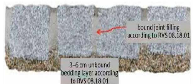
Figure 3. Sett pavement (paving elements) for the “composite” installation method (with cement-mortar joint filling) on an unbound (flexible) upper supporting layer
