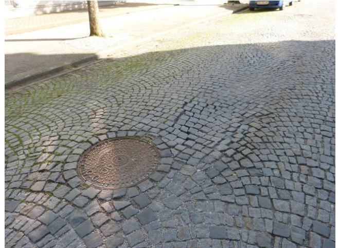
Figure 25. Rutting Source: Hrapović, 2025
